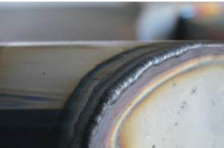
WELDED ELEMENT BEFORE PROCESSING
